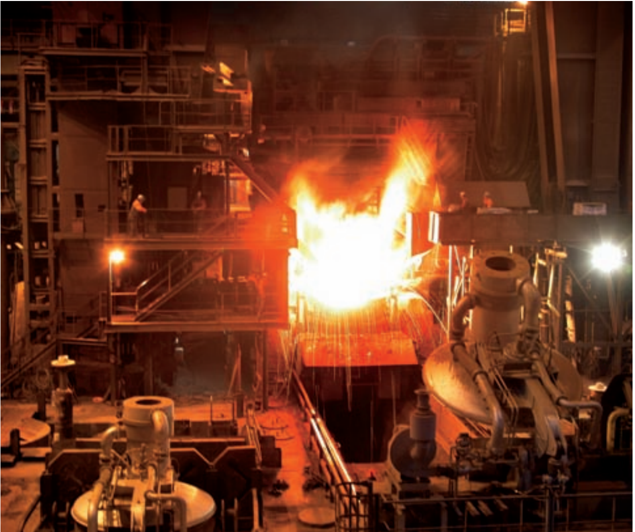
125 t UHP-Lichtbogenofen (LBO) | 125 t UHP Electric Arc Furnace (EAF)
